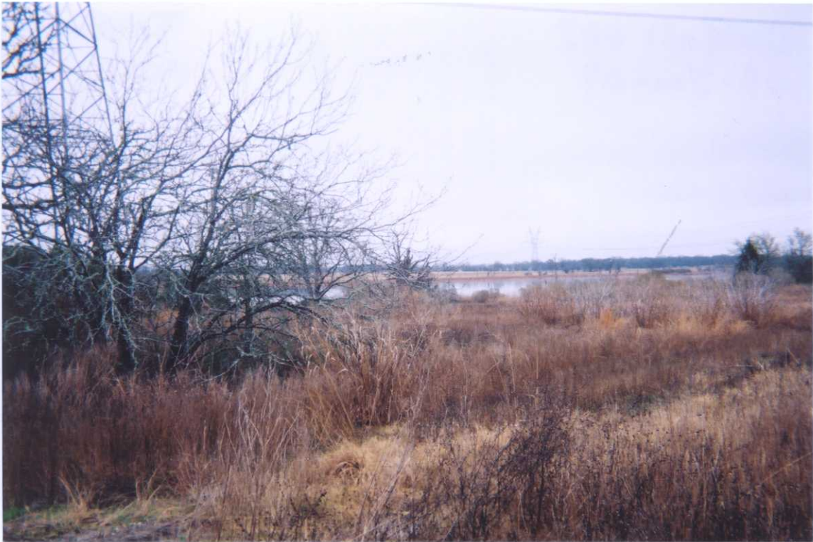
Outfall 003 Texas Municipal Power Agency Gibbons Creek Steam Electric Station Carlos, Texas
