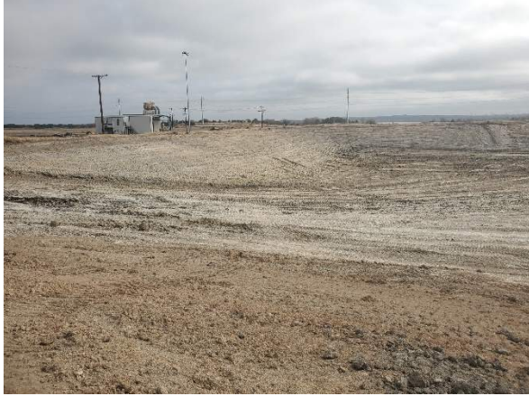
Figure 9: Scrubber Sludge Pond CCR Removal
