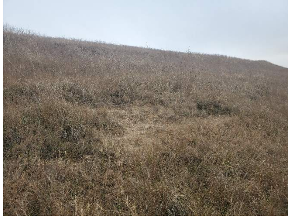
Figure 4: Side Slope Erosion
