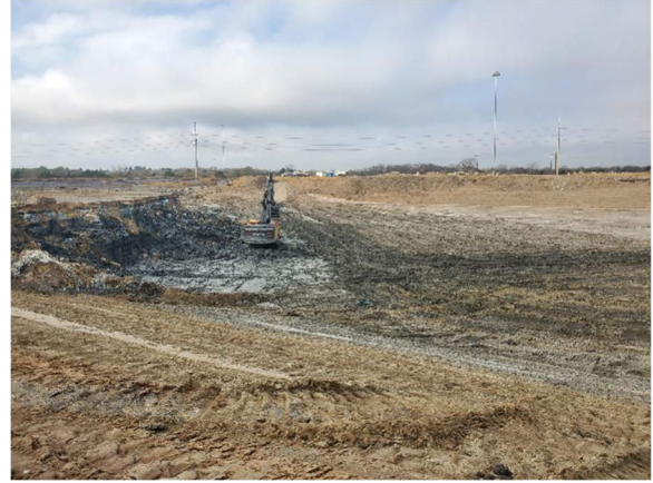
Figure 10: Scrubber Sludge Pond CCR Removal
