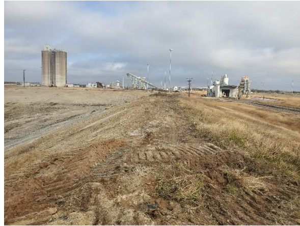
Figure 11: Scrubber Sludge Pond Containment Dike Status (typical)
