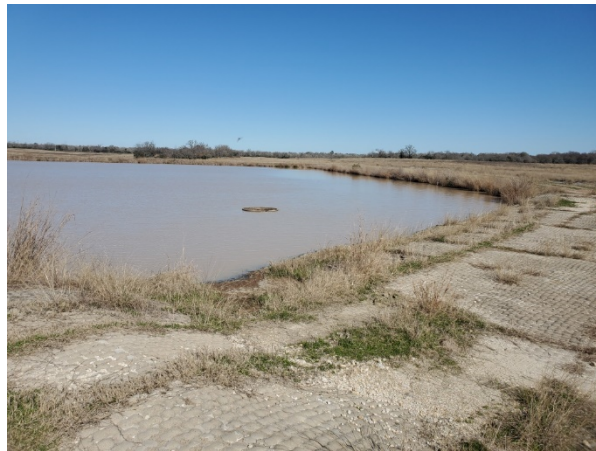
Figure 6: Settling Pond Cloudy
