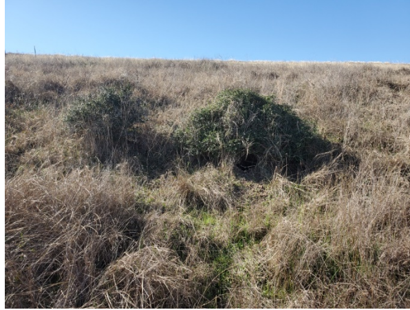
Figure 3: Typical Tree/Bush on Embankment
